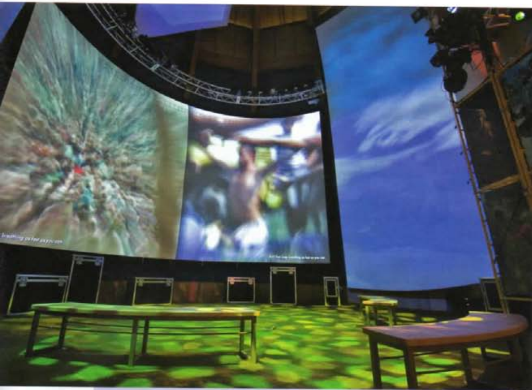
The museum's Festival Experience area uses six projectors blended to create one large image on a 40'x20' seamless, perforated curved screen, with a high-end audio system behind it. Three other projectors, complemented by small mirrors, fold the light into a vertical portrait mode and bounce video on to scrims above. The entire AV experience immerses viewers in a trip through the '60s.
